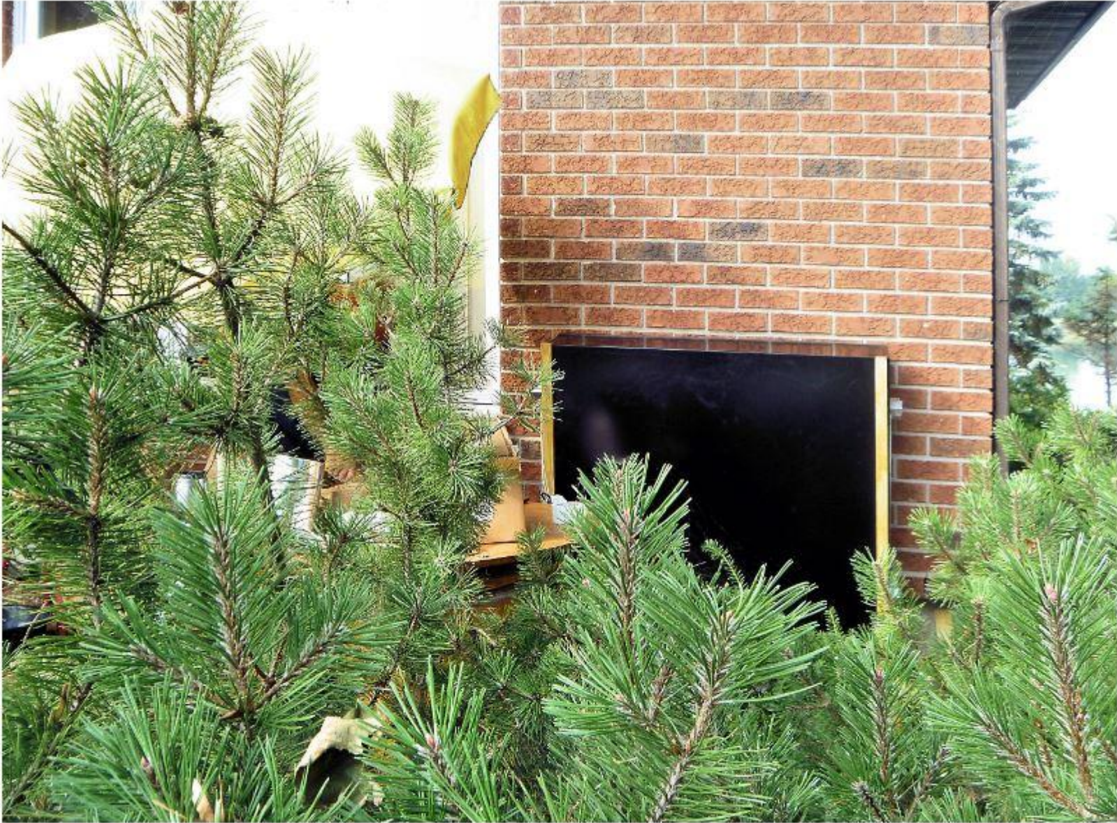
50 kW Air-heat exchanger transfers heat into the ground loop of the Test-bed system
